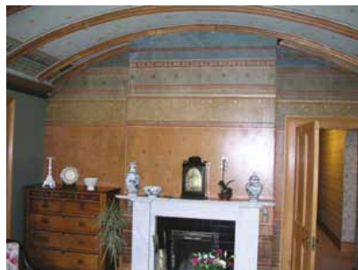
B Interior of Seaton Cottage, now Glenseaton Cottage, Bridge of Don after restoration. Courtesy of Bill Church.
