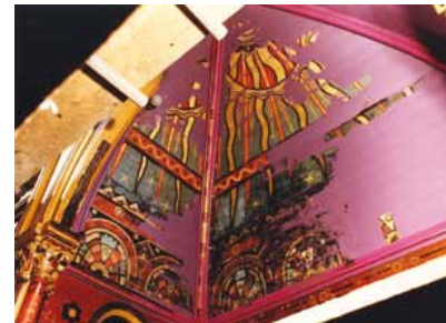
Fig 83 Pulpit Hood Underside, Dowanhill Church, revealing the original decoration beneath subsequent layers of purple paint. Courtesy of Historic Scotland.
